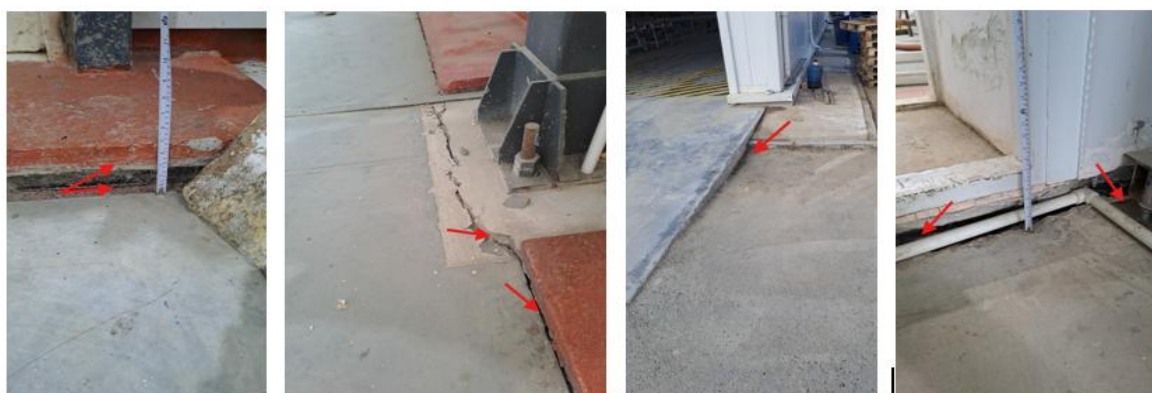
Figure 2 Foundation deformation
