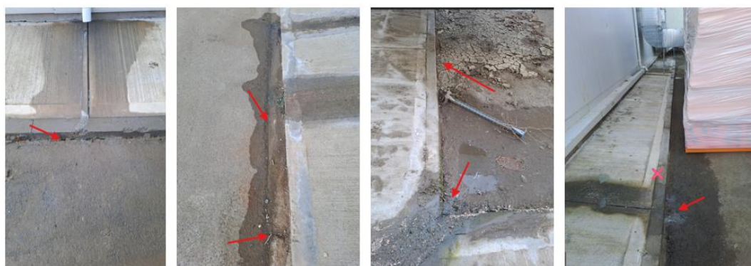
Figure 3 Infiltration of industrial and stormwater
